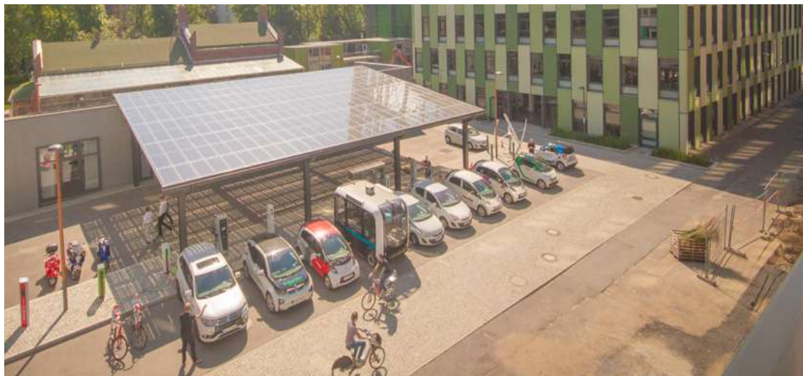
Figure 8: Mobility2Grid’s real-world laboratory: ZeeMo.Base innovative electric vehicle charging station.
